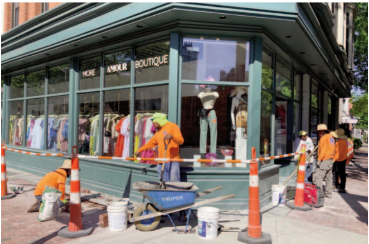
R&R Concrete for Elm City Properties replaces broken brick and stone along the sidewalk in front of shops More Amore and Book Trader.
