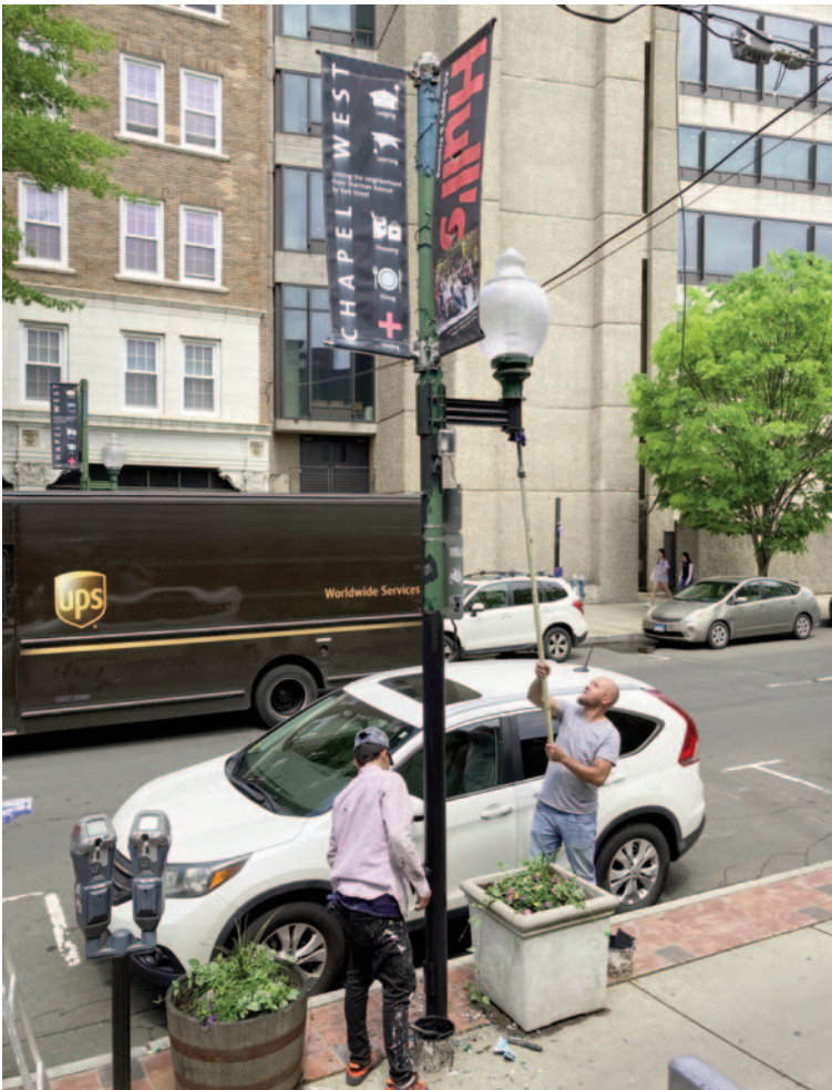
104 street banner poles on Chapel Street are given a new coat of black paint
