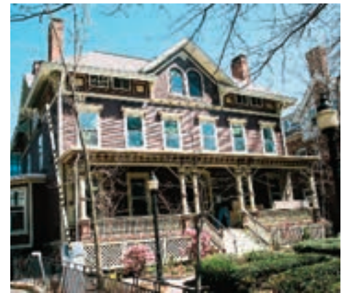
Yale University has completed the renovations of the former Inn at Chapel West . They have moved in the Yale Alumni Association to a second location there. The AYA will still remain in their Alumni House on York St. , as well. We are excited that they chose to locate in our district.
