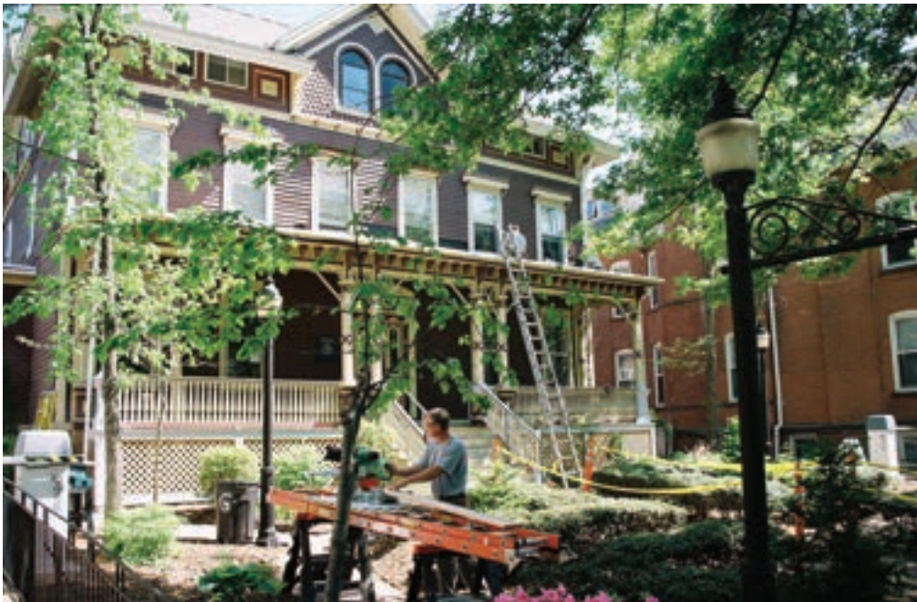
Renovations at AYA
