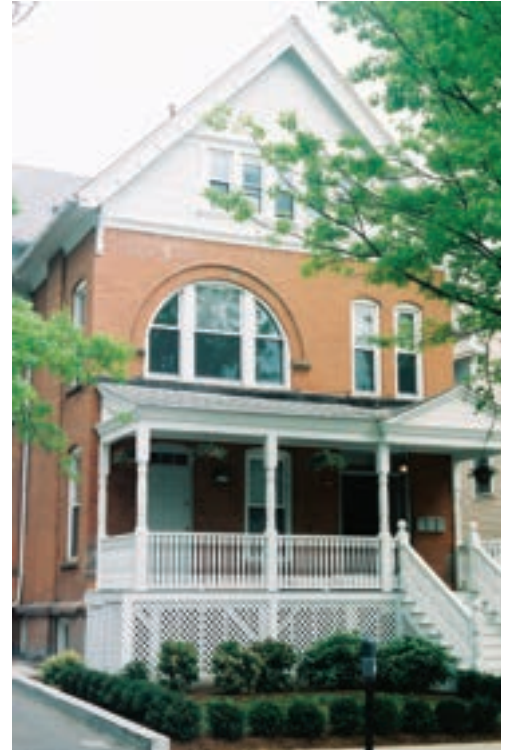
1195 Chapel St. with its brand new porch.
