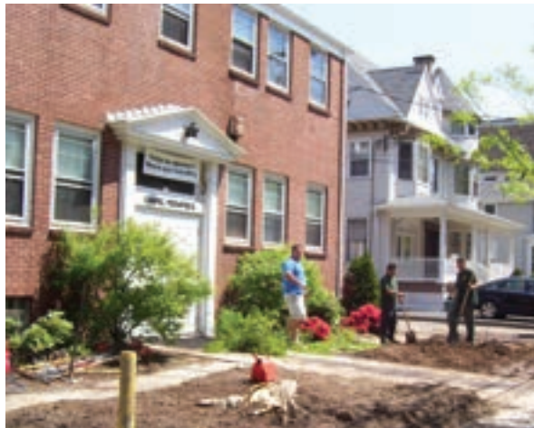
1441 Chapel St. landscaping
